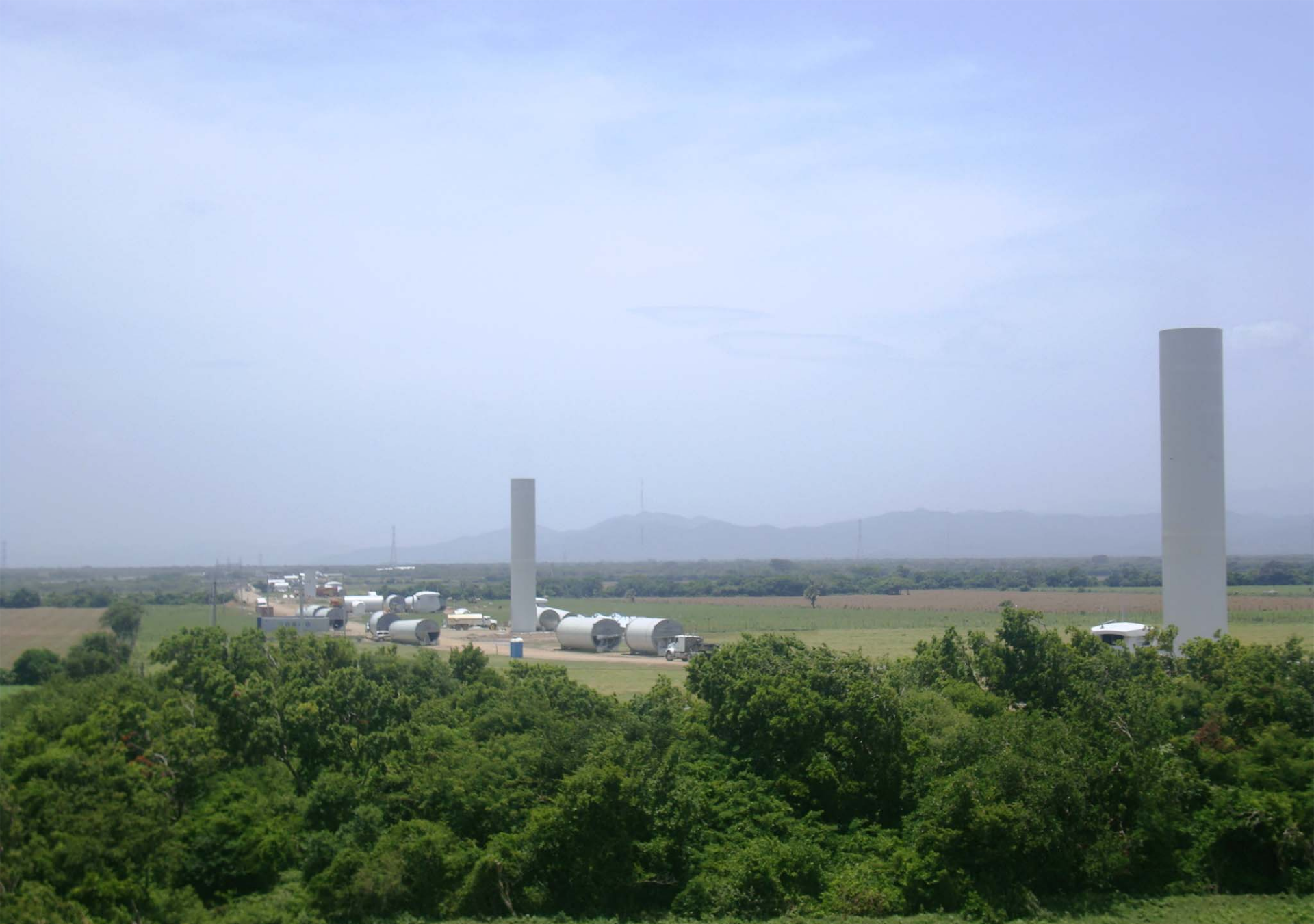
General view of erection works – La Mata
