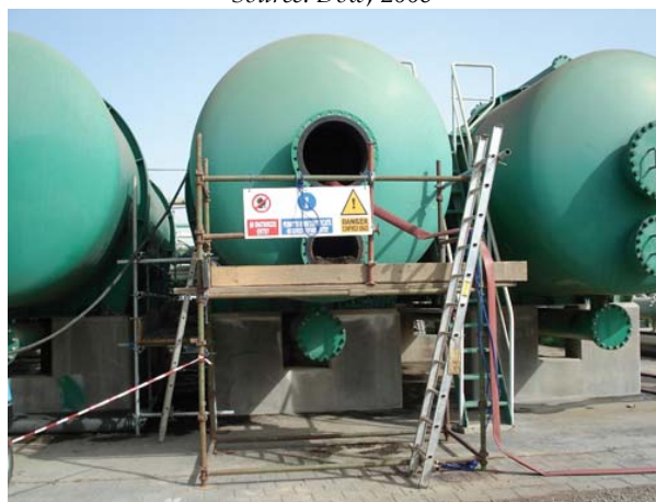
Figure 8-6 Horizontal Sand Filter Source: Dow, 2008
