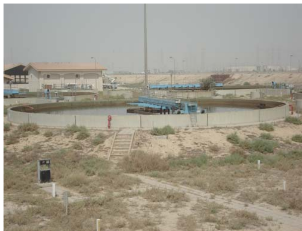
Figure 8-4 Aerators and Clarifiers Installed Directly in the Sand Base Source: Dow, 2008
