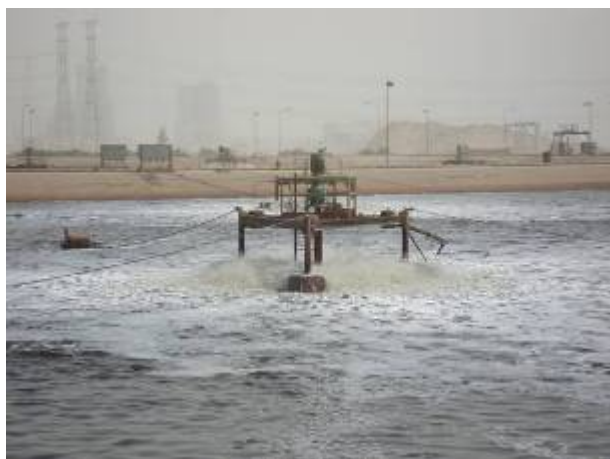
Figure 8-3 Surface Aerator Source: Dow, 2008
