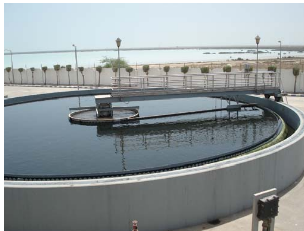
Figure 8-7 Secondary Clarifier Source: Dow, 2008
